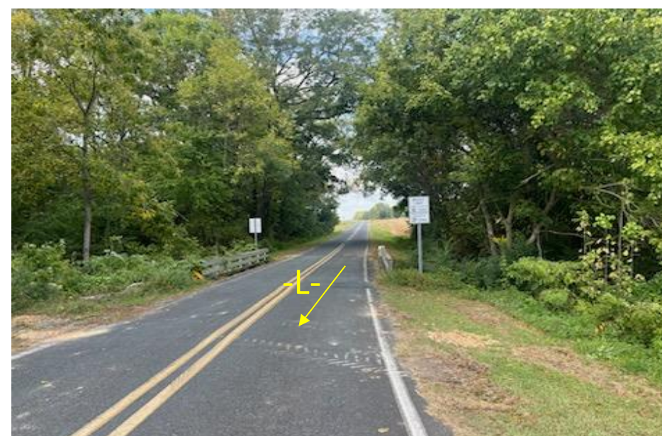
Bridge No. 890108 (Looking Northwest)
