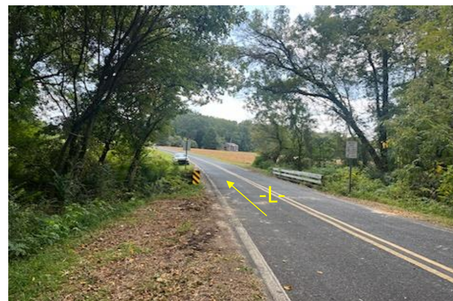
Bridge No. 890108 (Looking Southeast)
